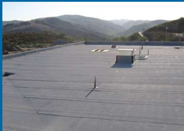
Diemer Filtration • Built Up Roof System • Yorba Linda, CA
