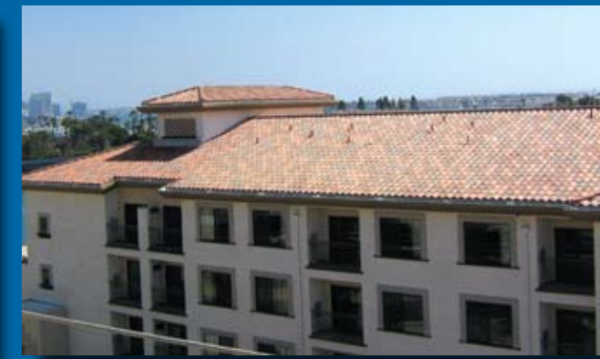
Homewood Suites • Clay Tile Roof System • San Diego, CA
