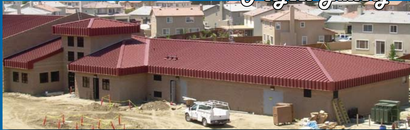
Hemet Water Treatment Plant • Standing Seam Metal Roof • Hemet, CA
