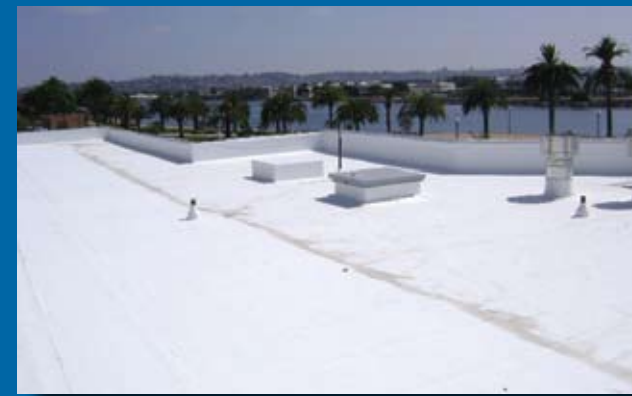
Courtyard Marriott • TPO Roof System • San Diego, CA
